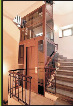
MRL LIFT ( MACHINE ROOM LESS )
